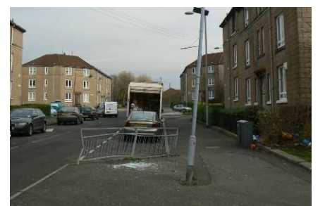
Damaged street furniture on Tobago Street
