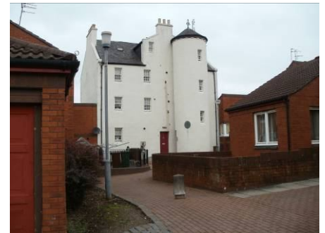
Chalmers Gate access to Chalmers Street
