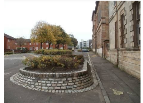
Former Tureen Street School
