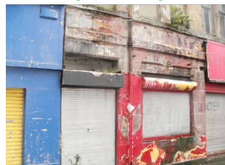
Derelict shops on Moncur Street
