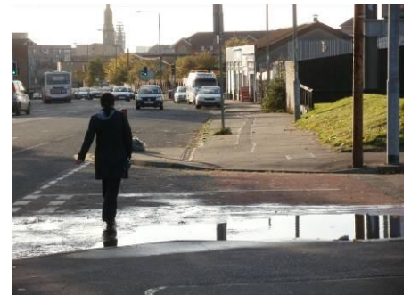
Ponding on Gallowgate
