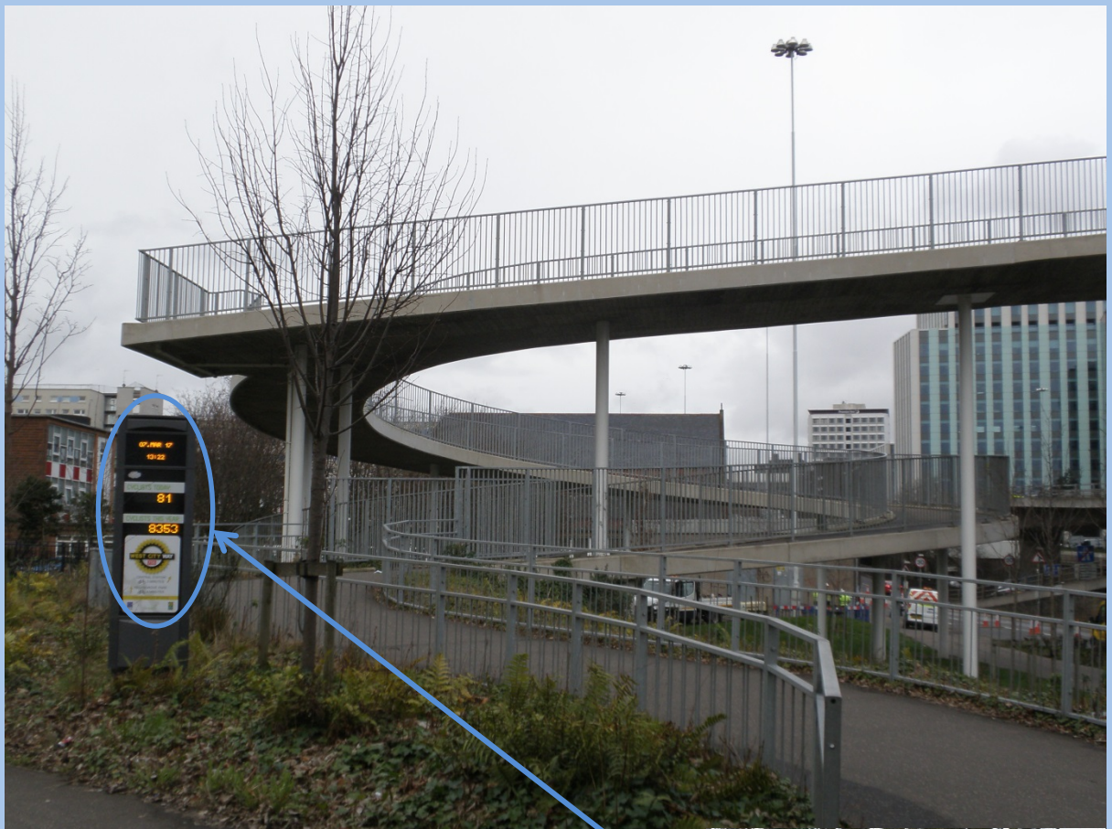
Figure 2a and 2b: The Anderston-Argyle Street Bridge and the cycle counter.
