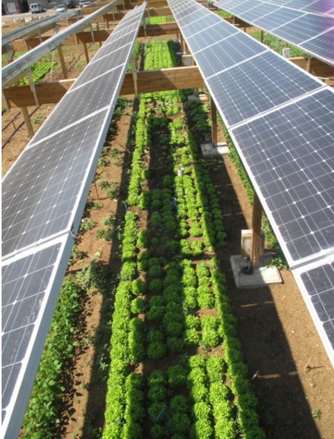
Photovoltaic (PV) Cells or Reflecting Mirrors for Concentrated Solar Power (CSP), provide important shade for crop growing in hot countries.
